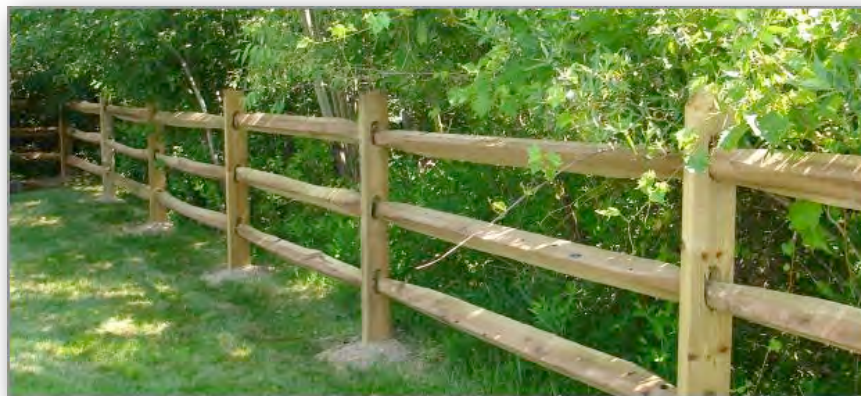
Wood Post and Rail Fence Example
