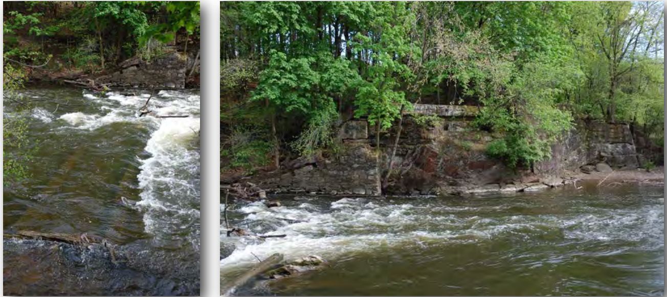
View of Timber Crib Dam and Infrastructure from Overlook
