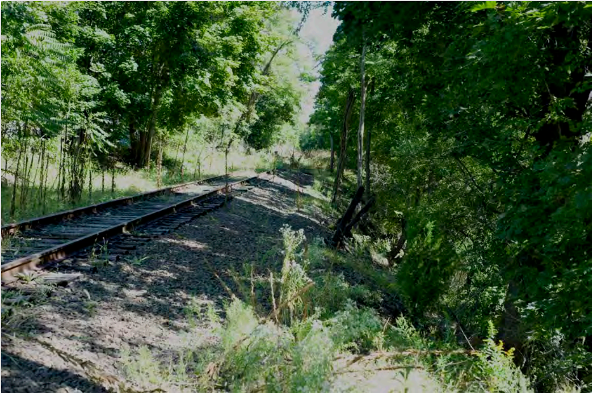
Existing Conditions View at Pinch Point (looking north)
