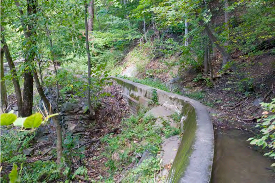
Existing Conditions View along Sucker Falls Raceway (looking south)
