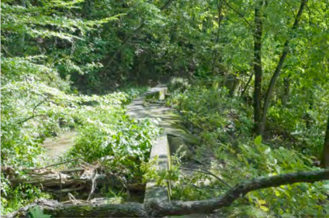
Existing Conditions View along Sucker Falls Raceway Wall (looking north)
