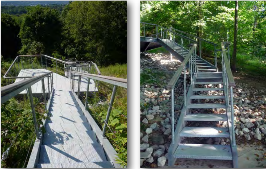
Outdoor Metal Staircase Examples (Mount Beacon Park)
